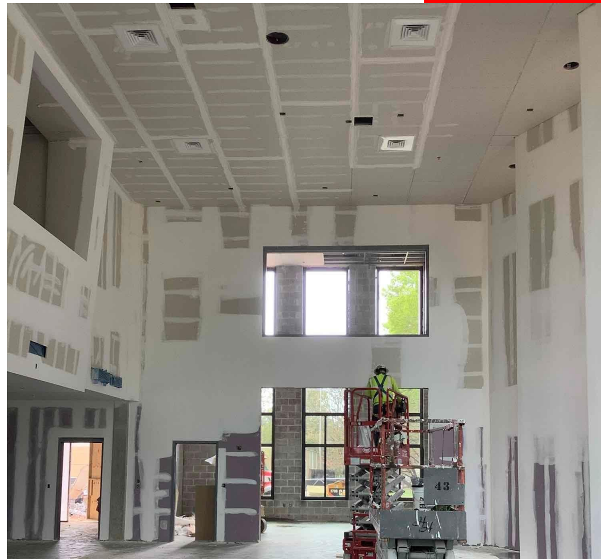
Gypsum Board Progress in Media Center Double Height Space
